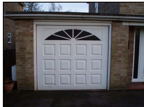
Garage attached to dwelling
